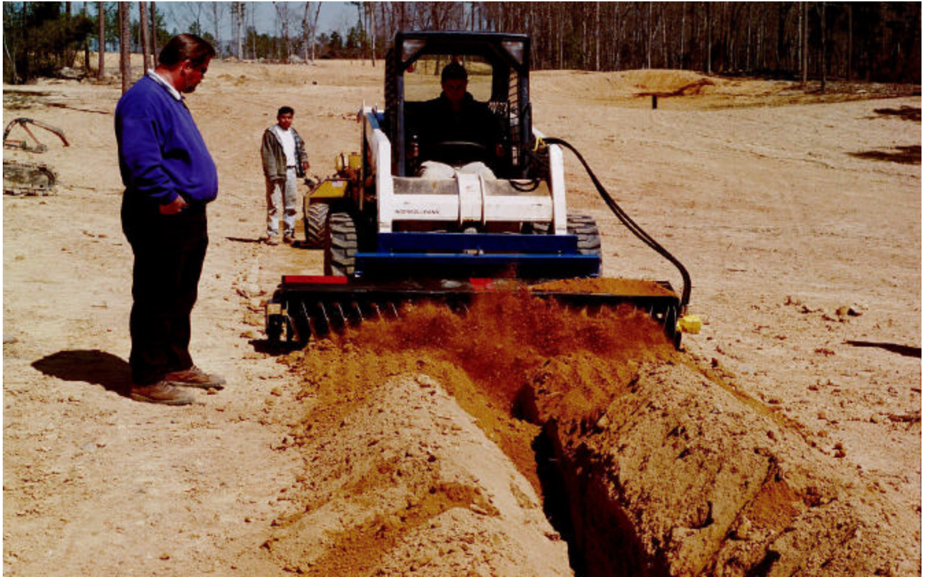
FIRST PASS OVER DITCH.
