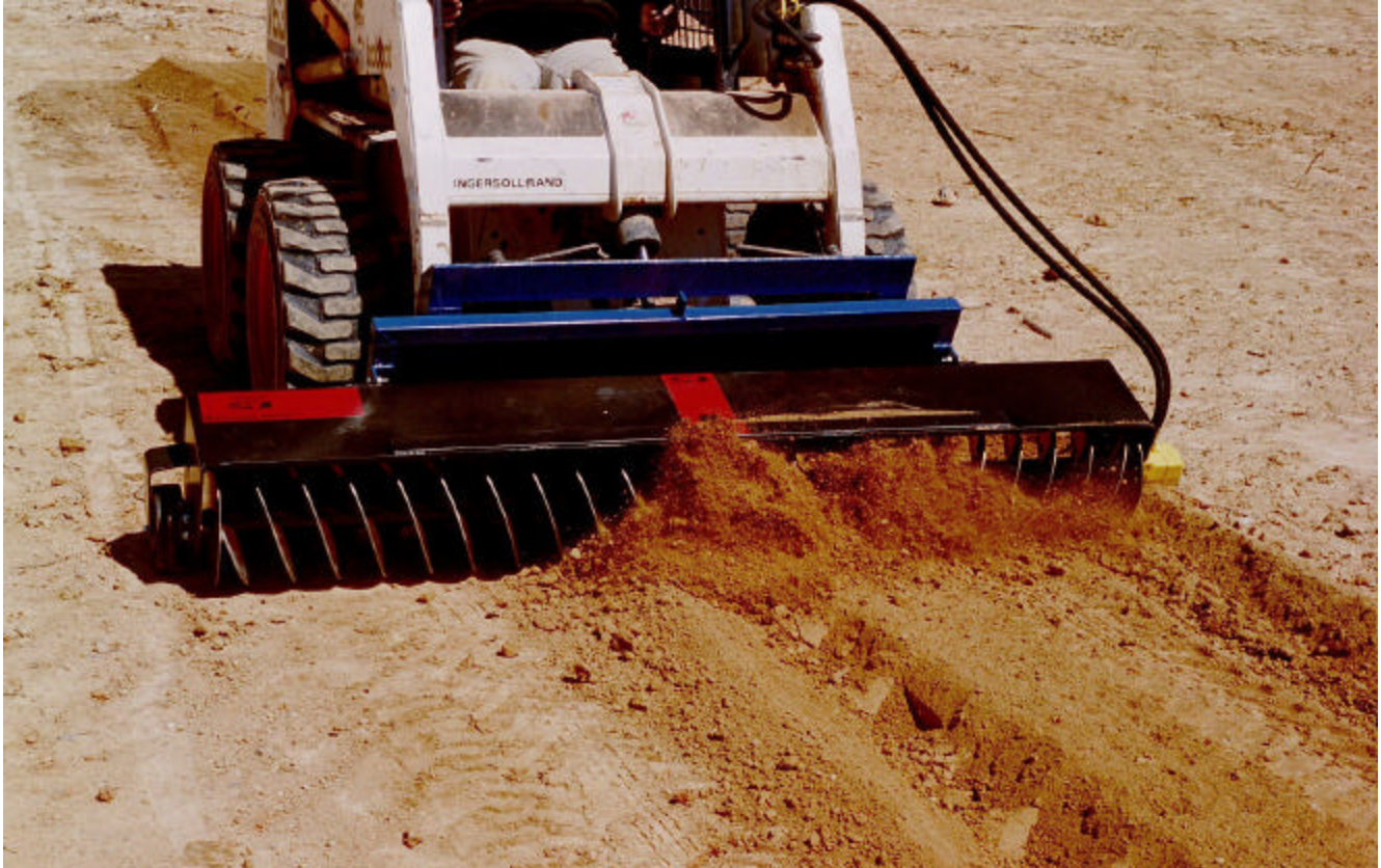
FINAL PASS AFTER TAMPING THE DITCH.
